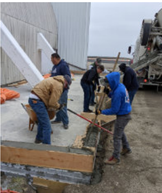
Pouring the foundation (K. Drewelow photo)
